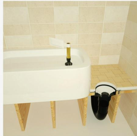
**8.** For easier insertion, apply lubricant to the tailpiece. Be sure to position the bathtub and tail piece in line with the drain body.
